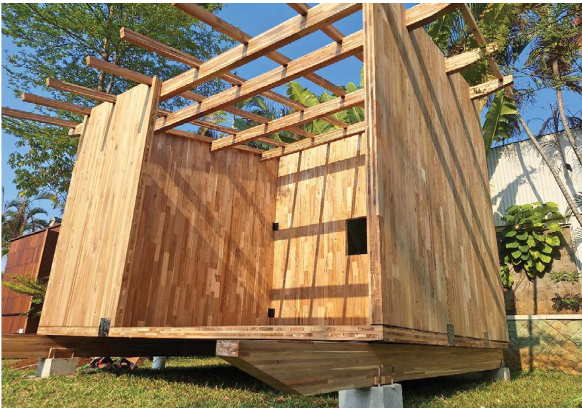
INCLT's first CLT unit with 3600 x 1200 x 75 panels, in South Jakarta
